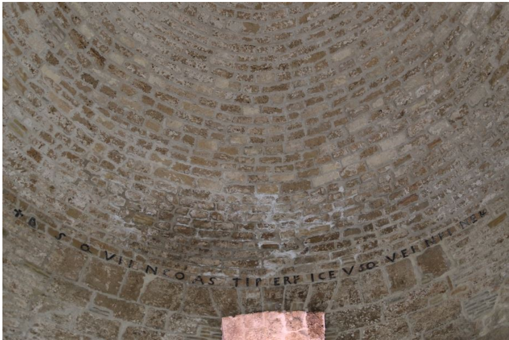
Fig. 3 - Inscriptions on the blocks at the base of the dome (photo by S.p.A.).
