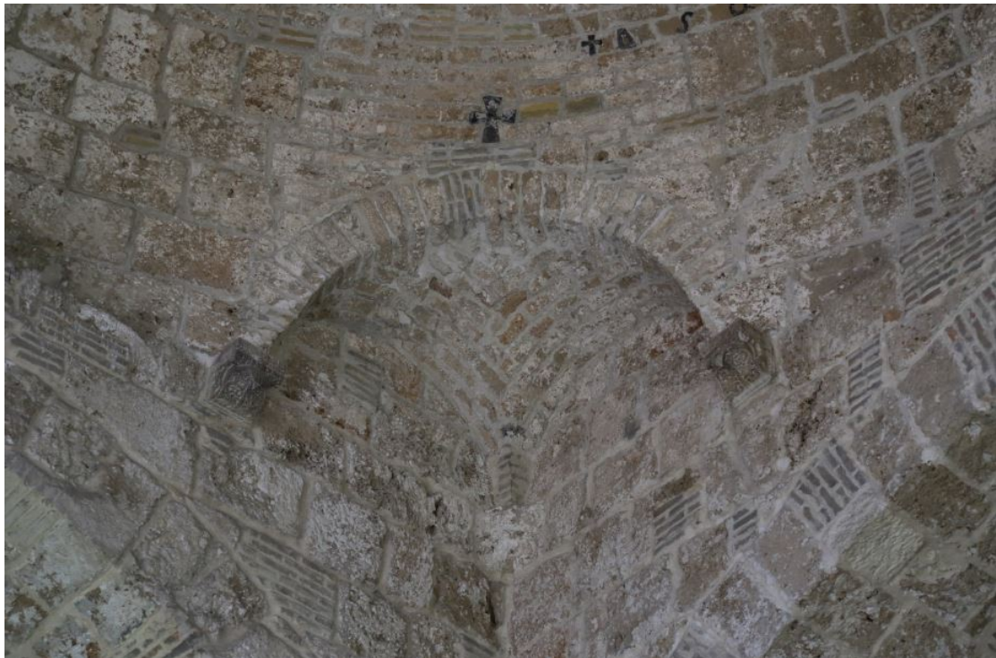
Fig. 2 - Detail of the connecting half cross vault between the round dome and the squared tholobate (photo by Unicity S.p.A.).
