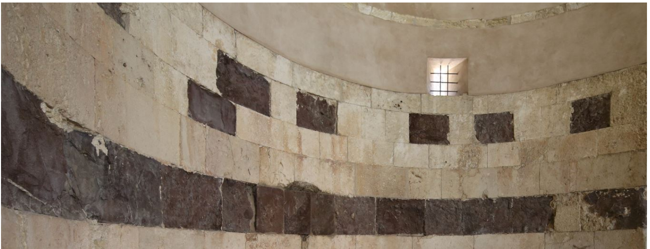
Fig. 3 - Detail of the building technique (photo by Unicity S.p.A.).
