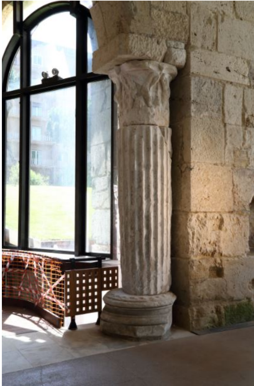
Fig. 2 - Reused architectural elements (base, column, capital) in the dividing wall of the right aisle of the eastern transept (photo by Unicity S.p.A.).
