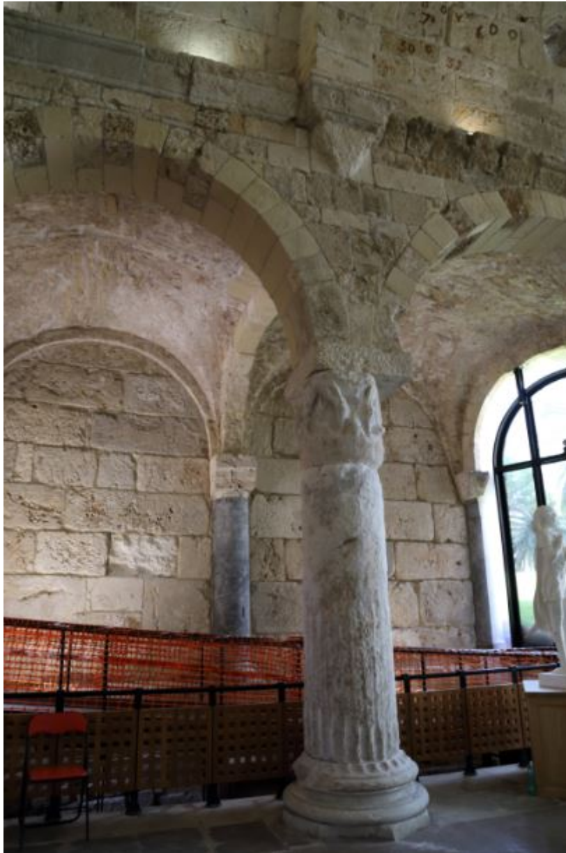
Fig. 3 - Reused architectural elements (base, columns, capitals) in the right aisle of the eastern transept (photo by Unicity S.p.A.).
