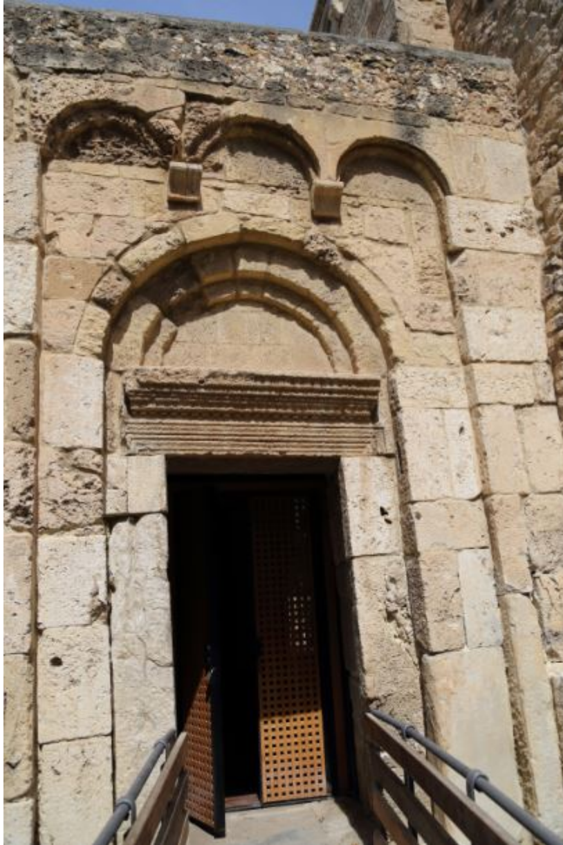
Fig. 2 - External entrance of the right nave of the eastern transept (photo Unicity S.p.A.).
