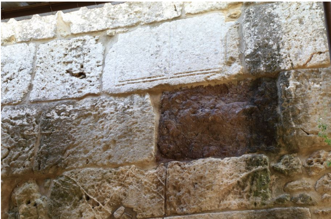
Fig. 1 - Funerary element with framed epigraphs redeployed outside the north wall of the western transept (photo by Unicity S.p.A.).
