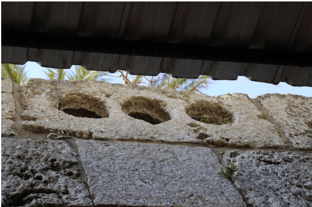
Fig. 1 - Ashlar with recesses for funeral urns, reused outside on the north wall of the western transept (photo by Unicity S.p.A.).
