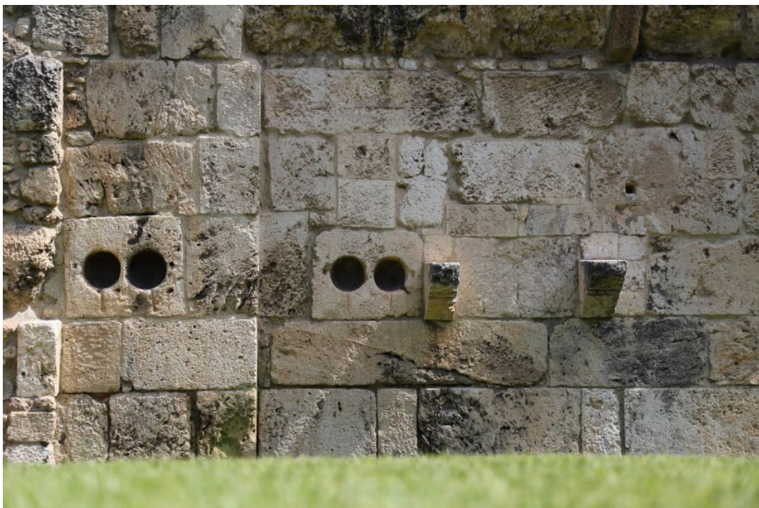
Fig. 3 - Ashlars with recesses for funeral urns, reused outside on the south wall of the eastern transept (photo by Unicity S.p.A.).
