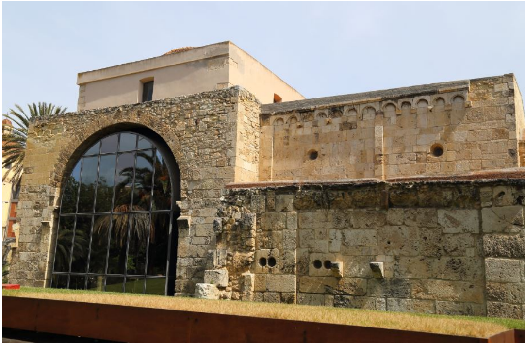
Fig. 1 - The domed structure and east transept seen from the south (photo by Unicity S.p.A.).
