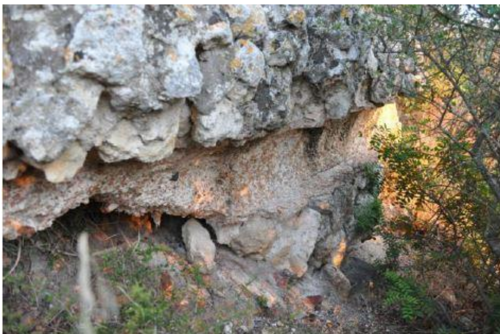
Fig. 2 - Stretch of the aqueduct (from FANTAUZZI, DE VINCENZO 2013, p. 3, fig. 3).
