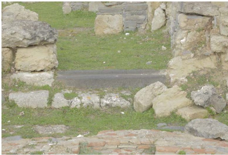
Fig. 6 - Threshold of the communicating access between the two churches, seen from the South (photo by Unicity S.p.A).
