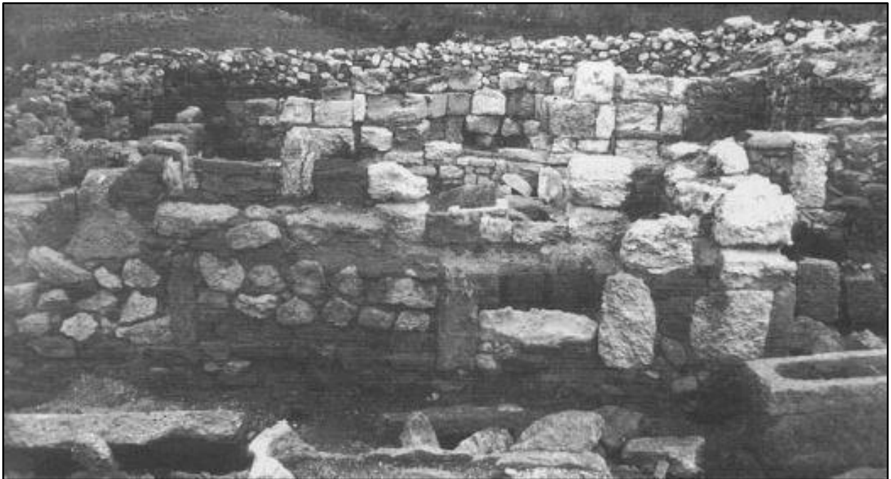
Fig. 4 - Wall in opus africanum in the corridor connecting space A and the funerary basilica. (from FANTAUZZI, DE VINCENZO 2013, p. 9, fig. 2).
