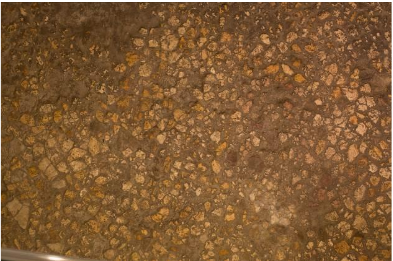
Fig. 1 - Dirt floor of the porticus (photo by Unicity S.p.A.).
