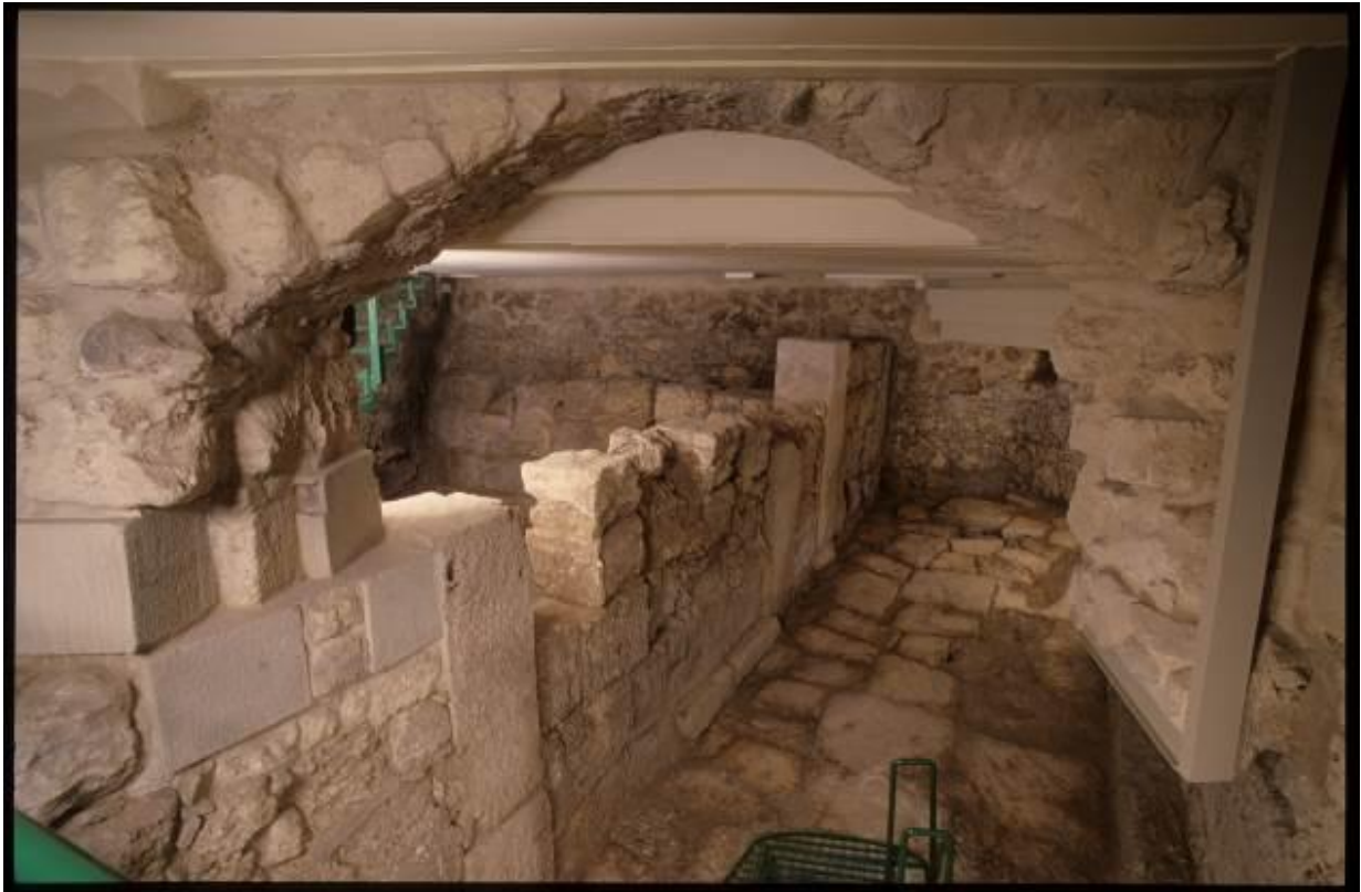
Fig. 2 - Frame wall closing the house to N-W obstructing access to the road. At the top, 17th century arch (photo by AFS).
