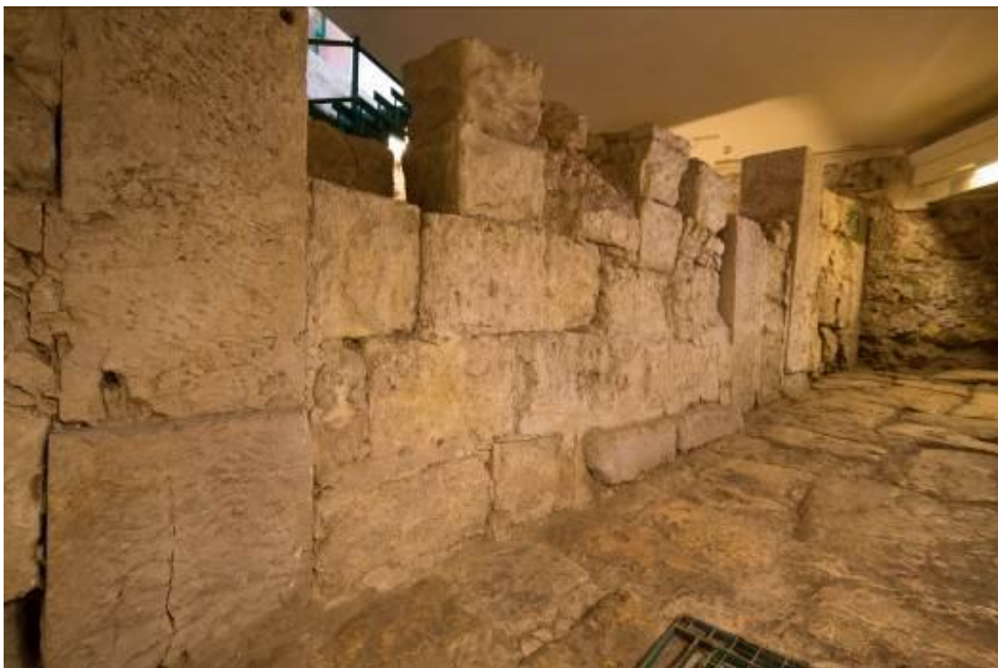
Fig. 1 - Wall in opus africanum (photo by Unicity S.p.A.).
