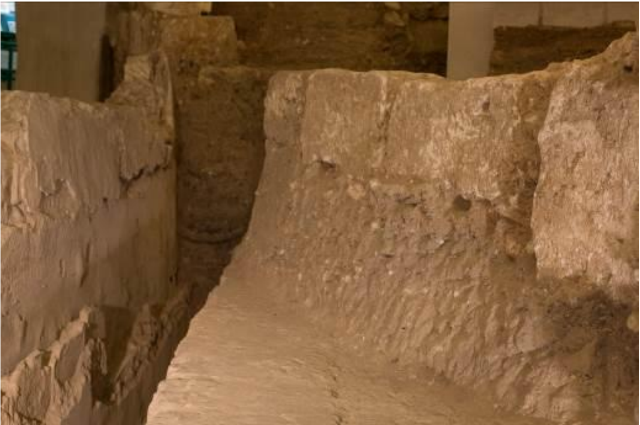
Fig. 1 - Wall structure of the building built on a thick layer of sediment. Its continuation stood on the shaved portico structures (photo by Unicity S.p.A.).
