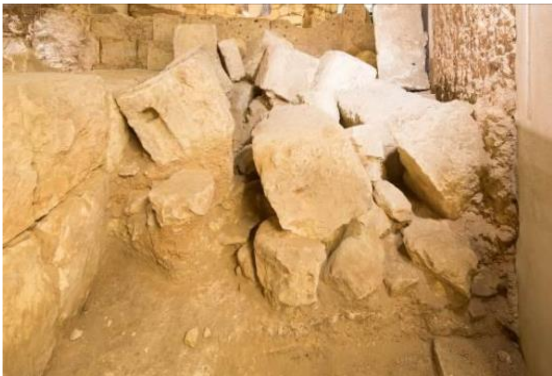
Fig. 4 - Blocks related to the II collapse on the left side of the transversal wall, standing on a layer of the previous collapse (photo by Unicity S.p.A.).
