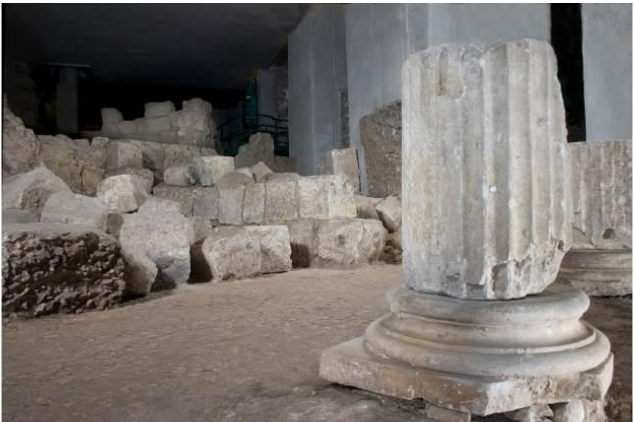
Fig. 1 - View of the portico with the second collapse in situ (photo by AFS).
