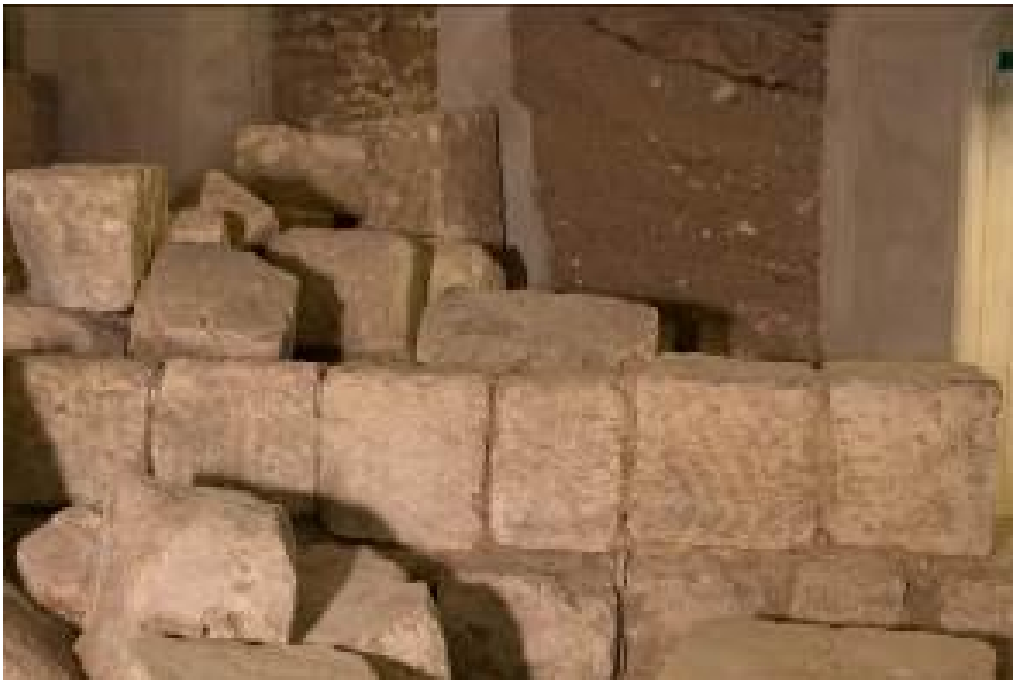
Fig. 1 - Transverse wall built with blocks reused recovered from the collapse and raised on a layer collapsed in the portico (photo by R. Martorelli).
