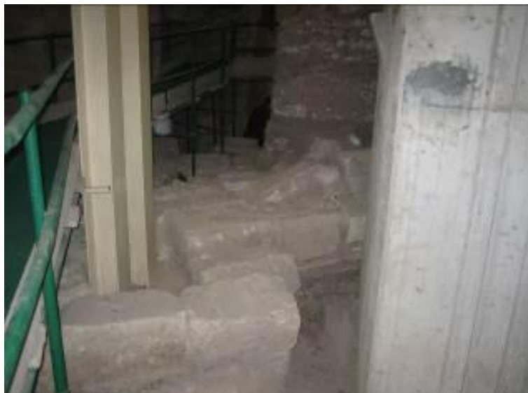
Fig. 3 - First collapse (photo by R. Martorelli).
