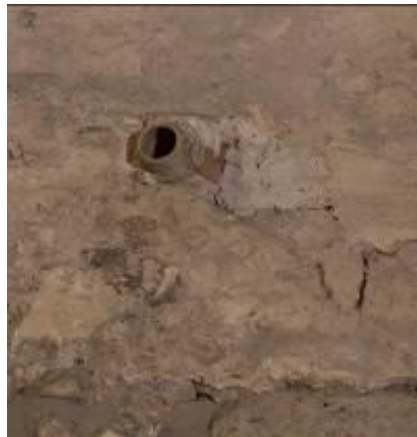
Fig. 3 - Fictile pipe (photo by Unicity S.p.A.).
