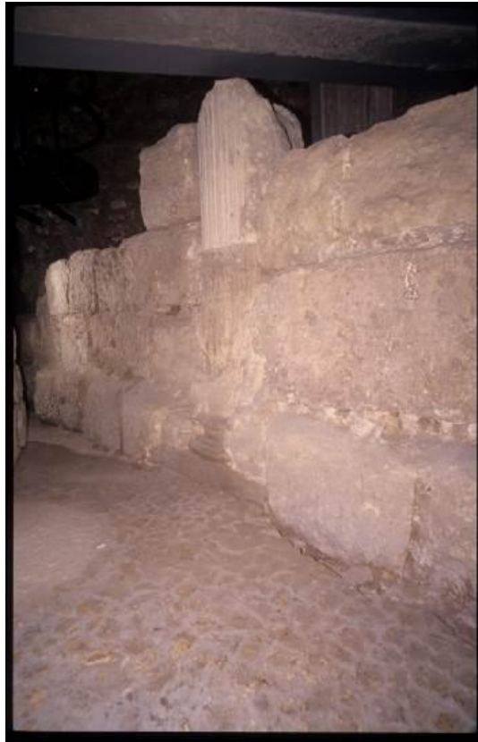
Fig. 3 - Column wrapped in shaped blocks (photo by AFS).
