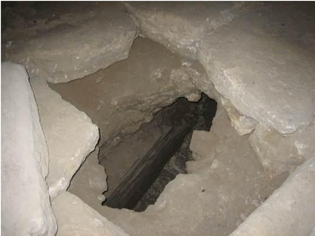
Fig. 1 - Sewer during digging operations (photo by Unicity S.p.A.).
