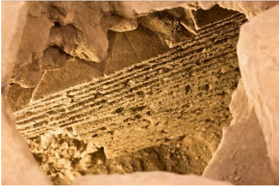
Fig. 2 - Inner sewer covering (photo by Unicity S.p.A.).
