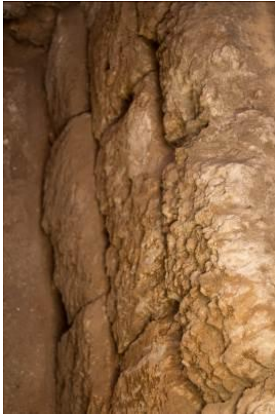
Fig. 2 - Ashlar blocks covering the sanctuary podium (photo by Unicity S.p.A.).
