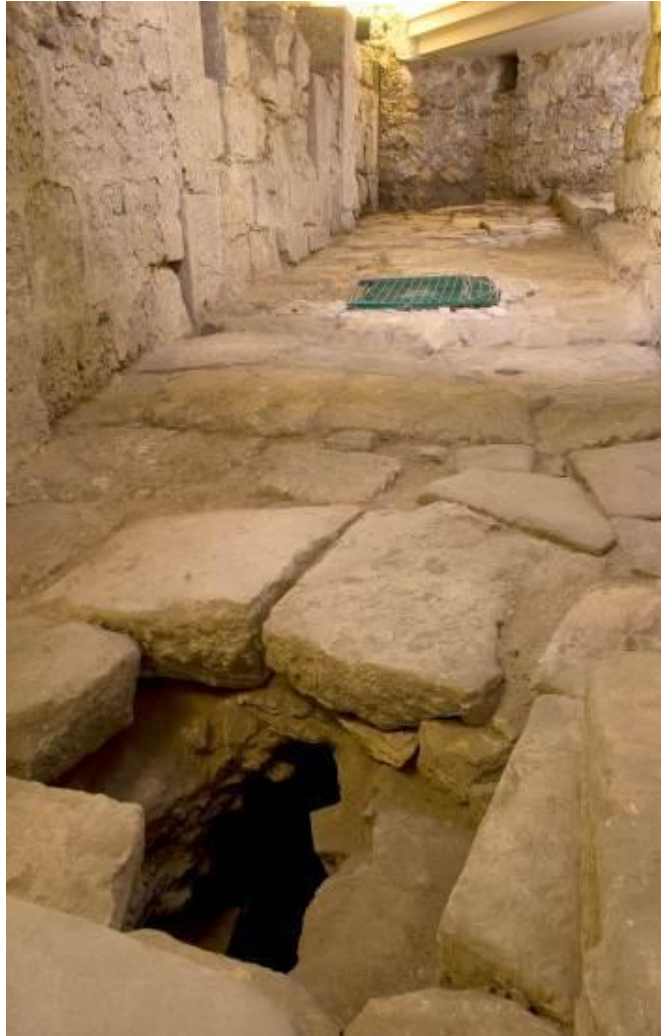
Fig. 1 - Sewer inspection pit, open on the paved road (photo by Unicity S.p.A.).
