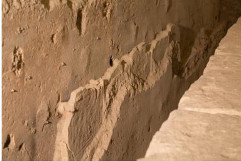
Fig. 6 - Hamatae tiles at the back of the colonnade (photo by Unicity S.p.A.).
