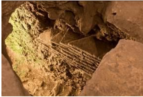
Fig. 3 - Stretch of sewer partly dug in the rock and partly built with brick fragments (photo by Unicity S.p.A.).
