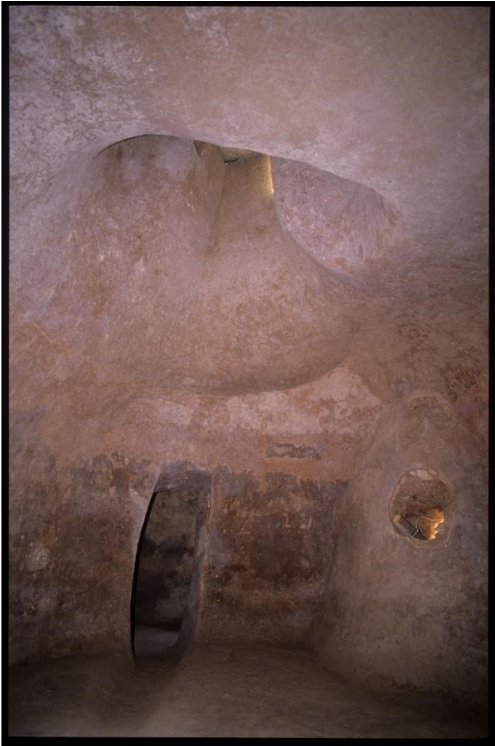
Fig. 5 - Cistern placed under the area with the raised floor (photo by AFS).
