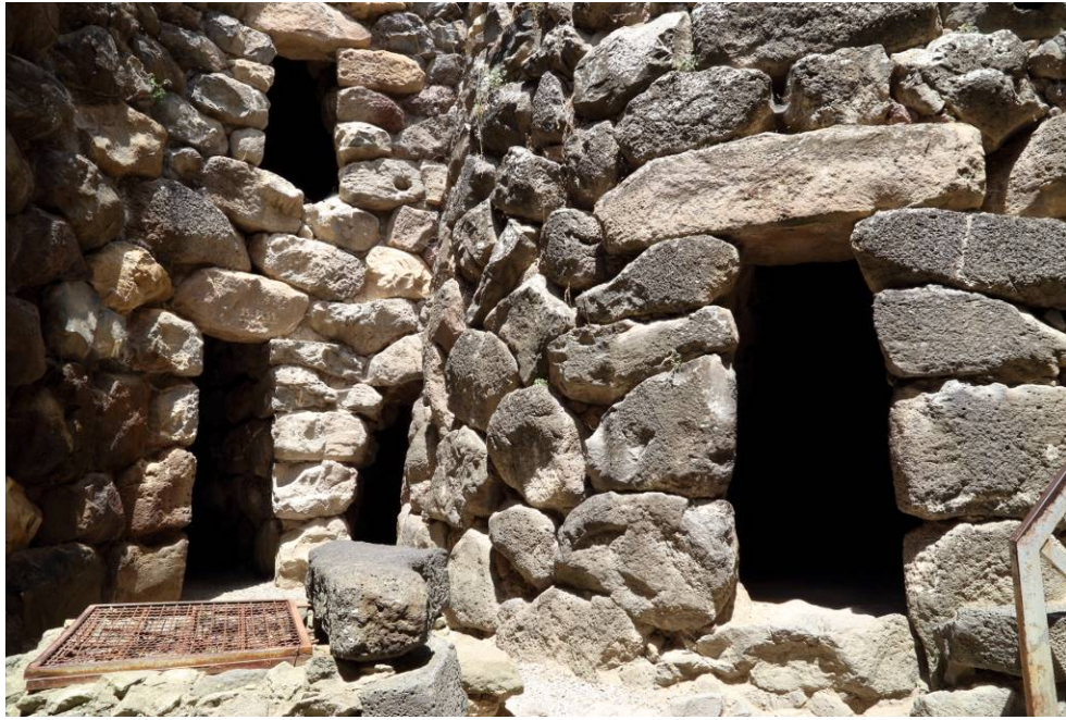
Fig. 2 - Right, the keep entrance (photo by Unicity S.p.A.).
