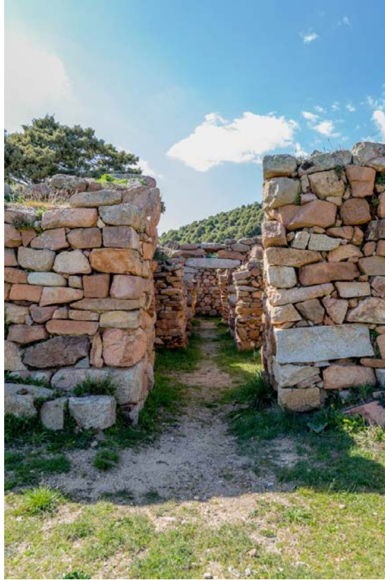
Fig. 2 - Detail of the entrance corridor to room A (photo by Unicity S.p.A.).
