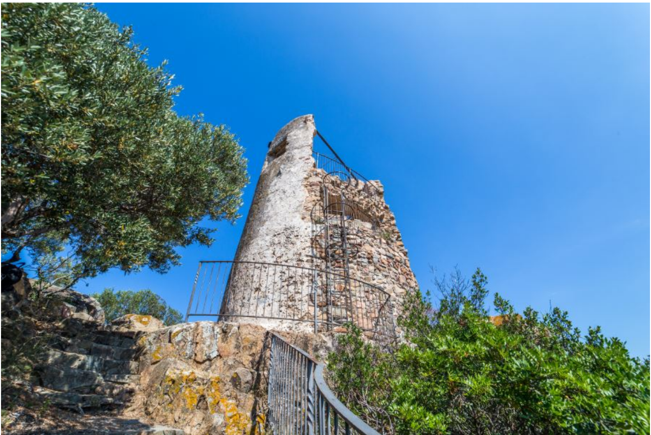
Fig. 5 - The tower of San Gemiliano seen from the east (photo by Unicity S.p.A.).
