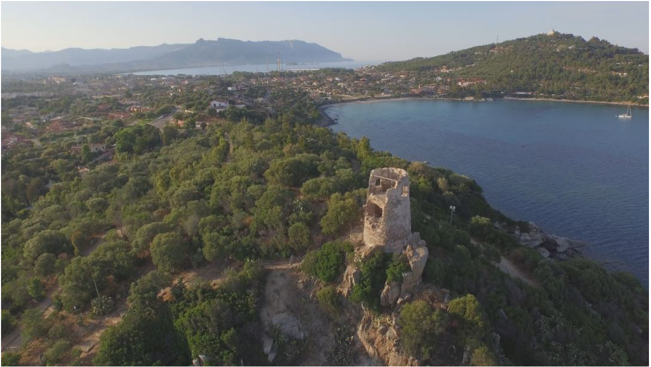
Fig. 3 - In the foreground the tower of S. Gemiliano; to the top right the Lighthouse of Capo Bellavista (photo by Unicity S.p.A.).
