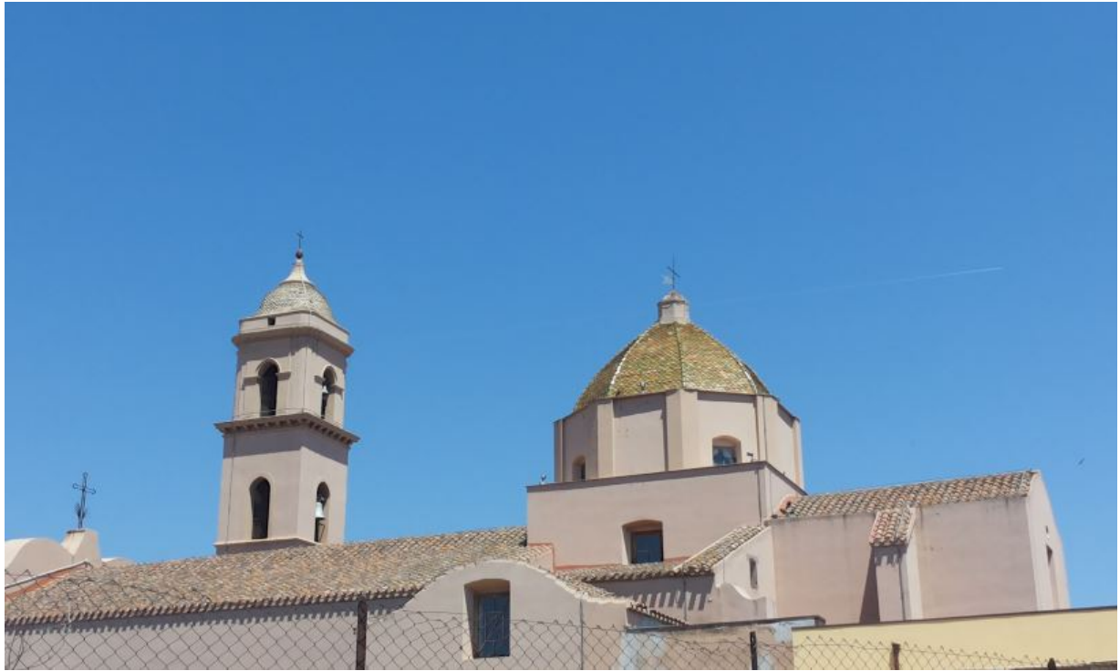
Fig. 2 - The church of S. Andrea seen from the outside (photo M.G. Arru).
