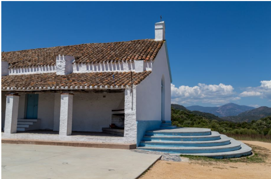
Fig. 4 - Portico with secondary entrance and fireplace (photo Unicity S.p.A.).
