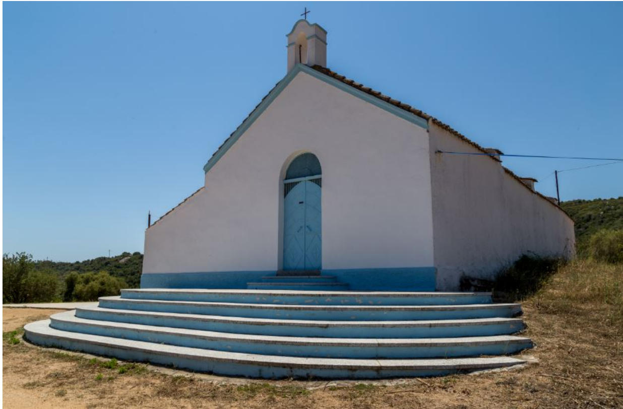
Fig. 2 - The main facade of the church of San Salvatore (photo Unicity S.p.A.).
