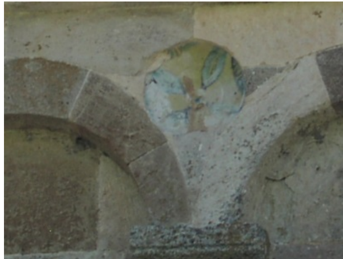
Fig. 3 - Detail of a ceramic bowl on the western side of the church of San Nicola di Trullas (photo by Unicity S.p.A.).
