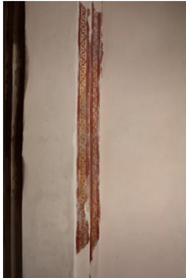
Fig. 2 - Details of painted decoration on the side walls (photo by Unicity S.p.A.).
