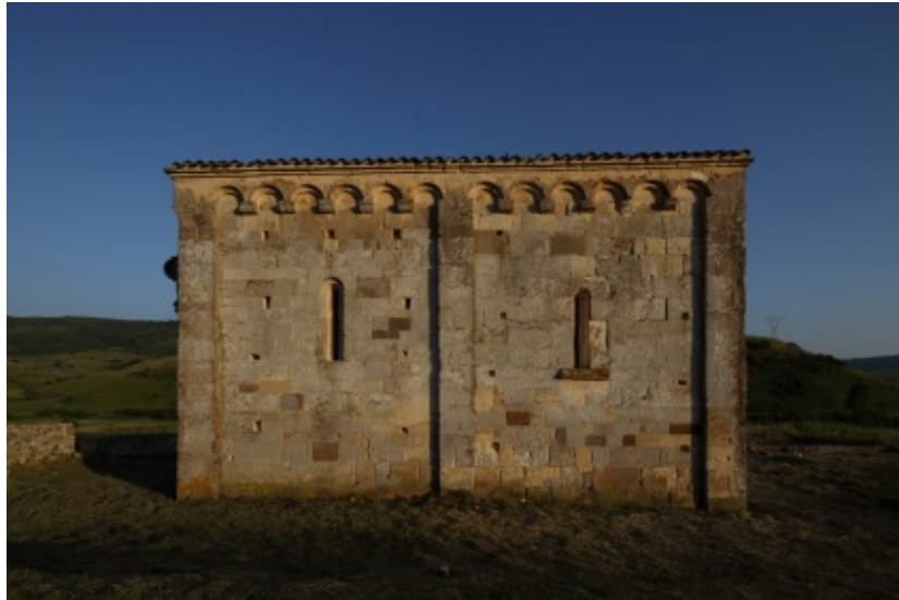
Fig. 2 - Northern Side (photo by Unicity S.p.A.).
