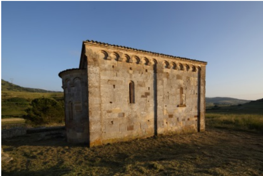
Fig. 1 - Northern Side (photo by Unicity S.p.A.).
