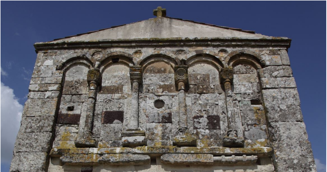
Fig. 2 - The upper part of the façade (photo by Unicity S.p.A.).
