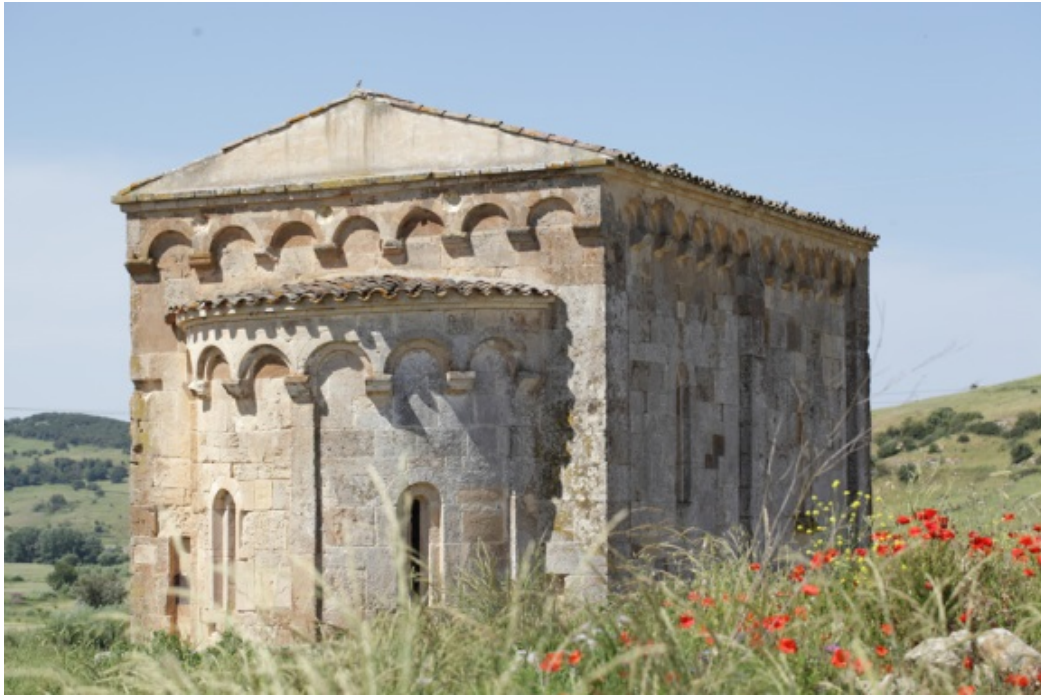
Fig. 2 - The church apse (photo by Unicity S.p.A.).
