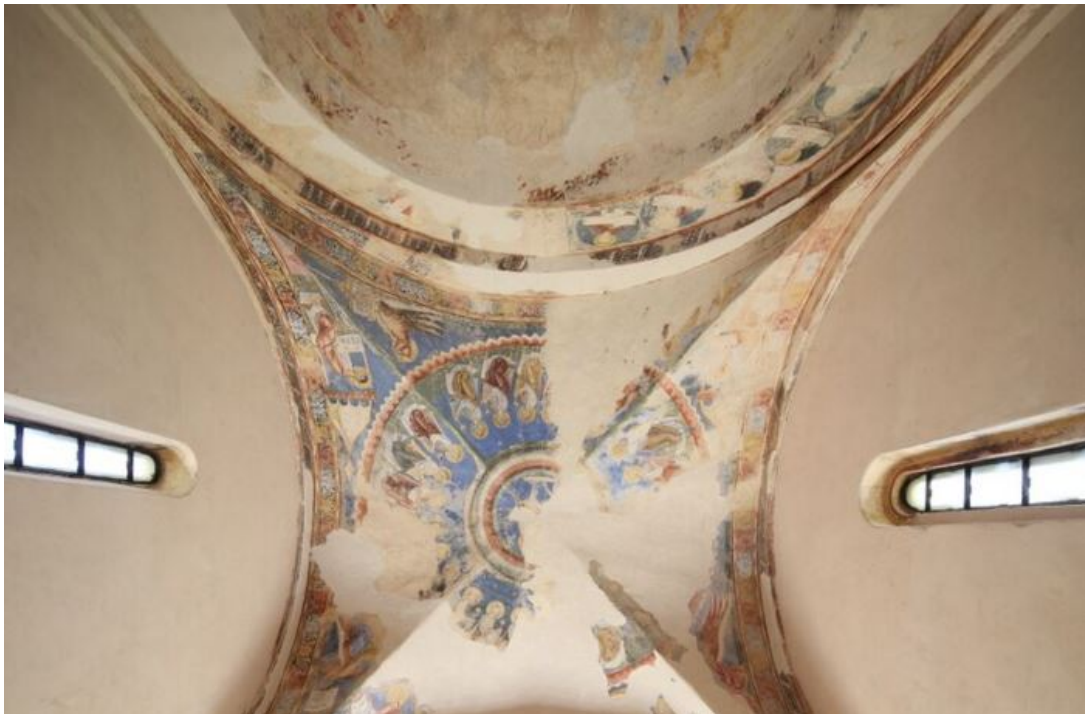
Fig. 3 - The cross vault of one of the bays (photo by Unicity S.p.A.).
