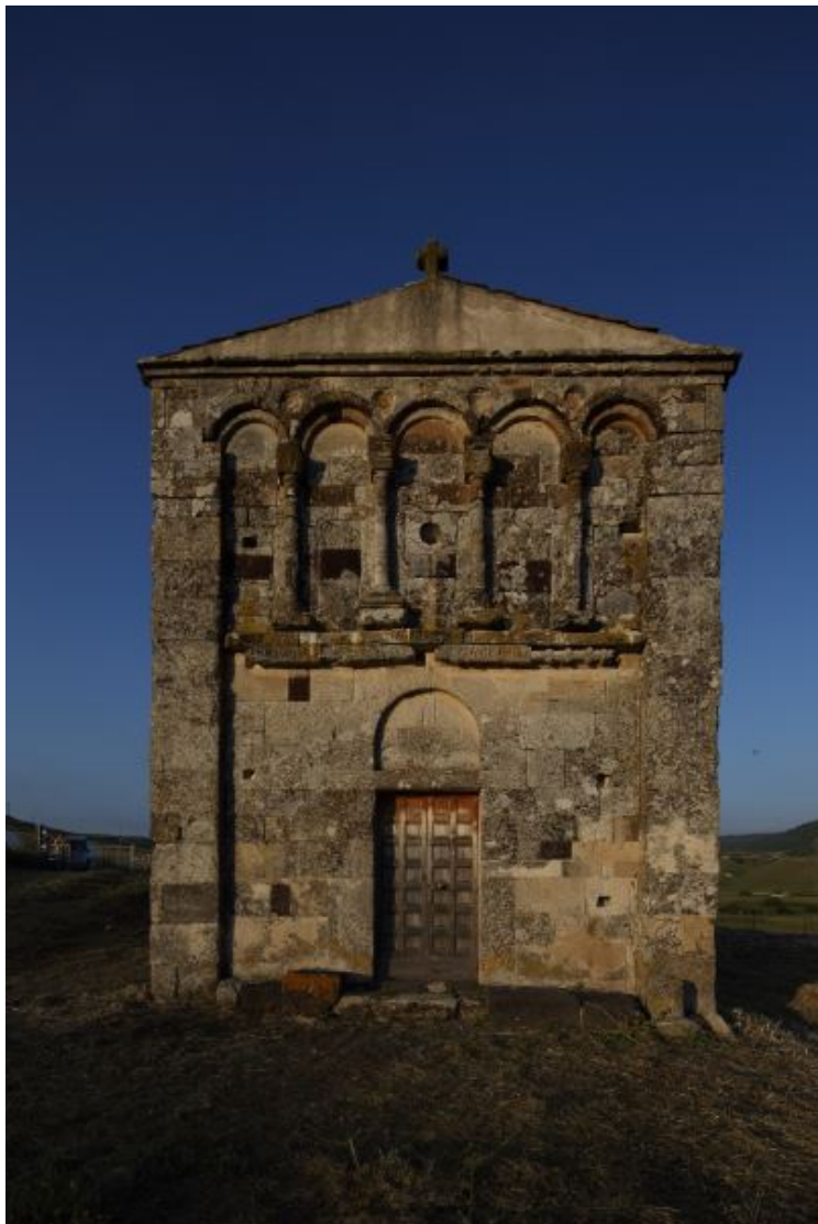
Fig. 1 - The façade of the church of S. Nicola di Trullas (photo by Unicity S.p.A.).
