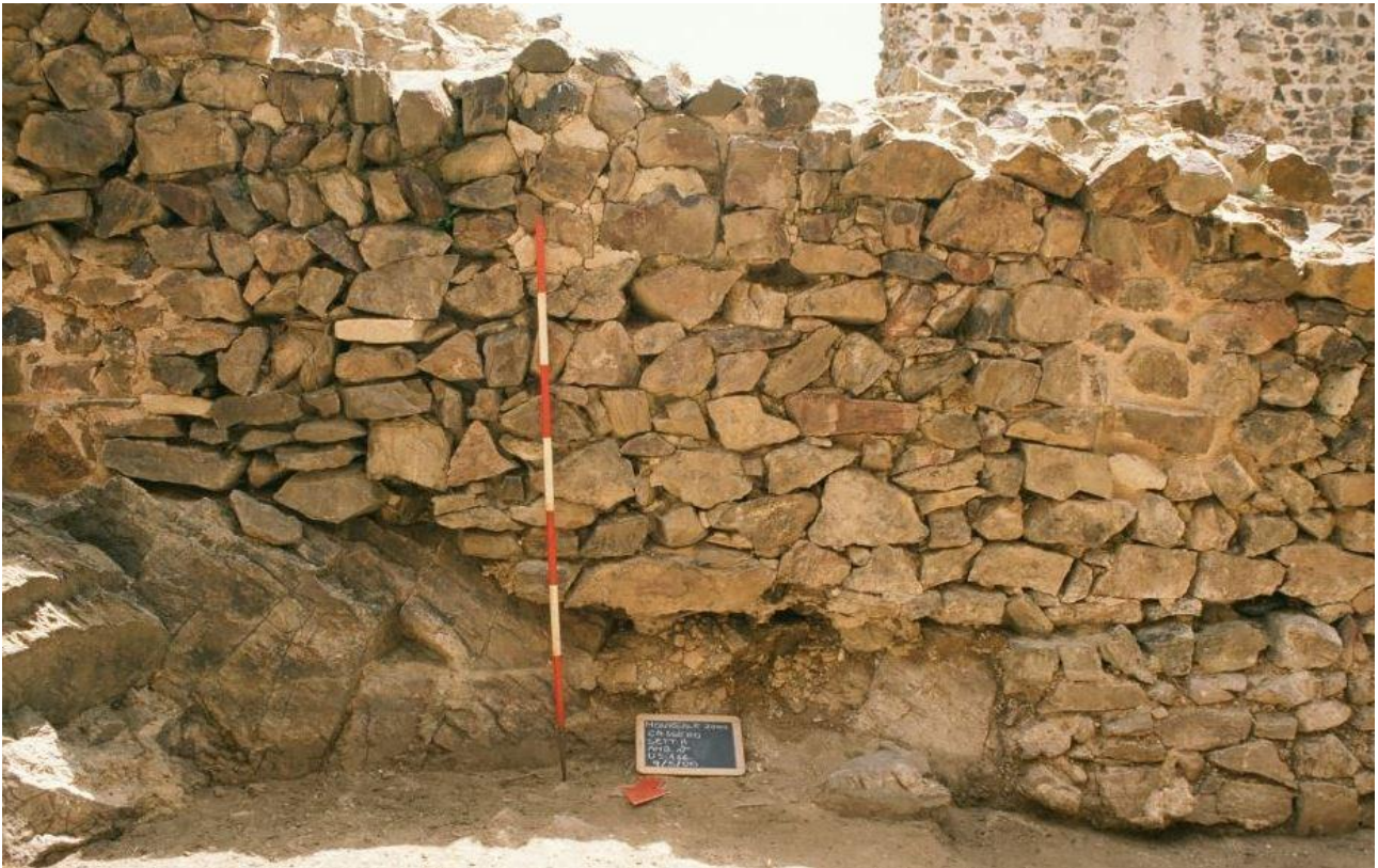
Fig. 2 - Wall building inside the theta room (photo by R. Bordicchia).
