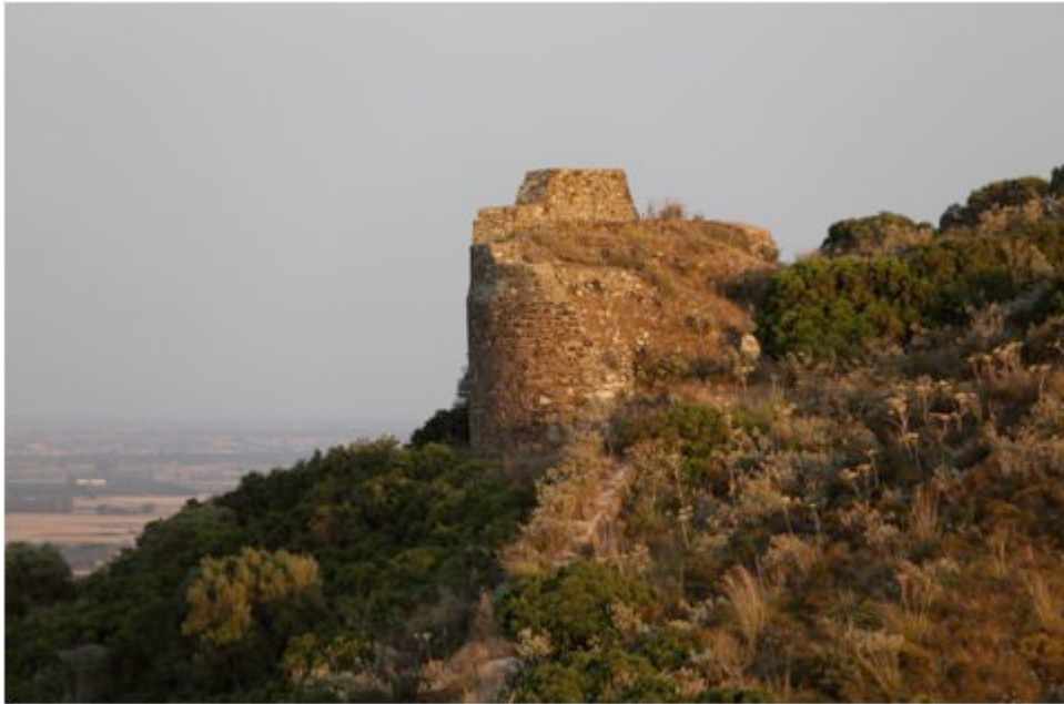
Fig. 4 - One of the semi-circular towers of the walls of the village (photo by Unicity S.p.A.).
