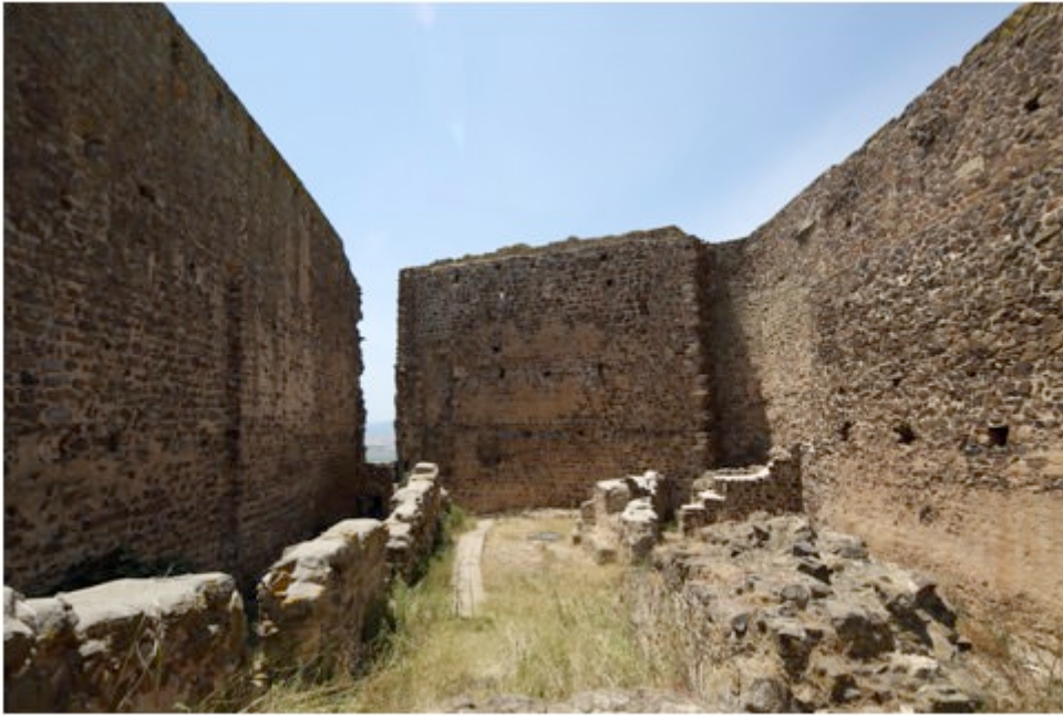
Fig. 13 - The interior of the castle from the East. The holes for housing the wooden beams can be seen on the walls (photo by Unicity S.p.A.).
