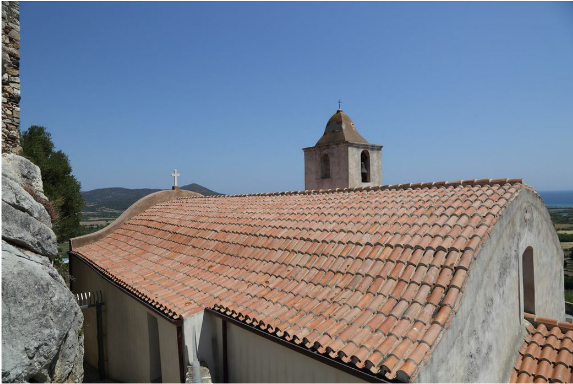
Fig. 3 - Posada, the church of Sant' Antonio Abate seen from the south west (photo by Unicity S.p.A.).
