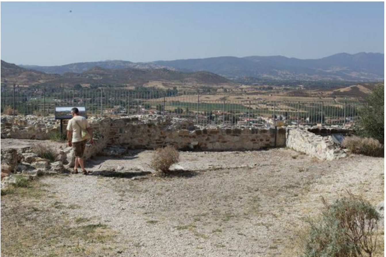
Fig. 2 - Detail of the wall crests which define the structure of the parade ground (photo by E. Dirminti).
