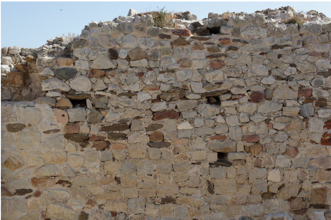
Fig. 3 - Holes housing wooden beams, arranged vertically (photo by Unicity S.p.A.).
