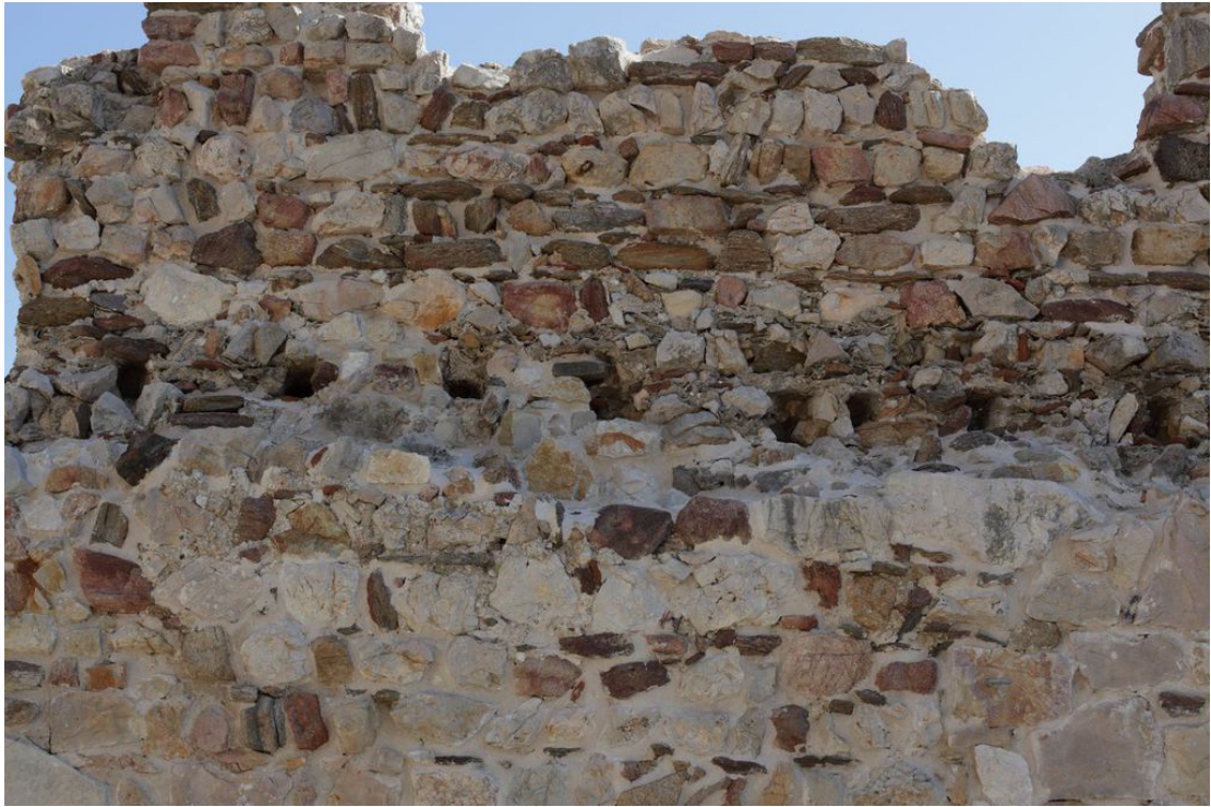
Fig. 4 - Housing holes arranged horizontally, for the supporting beams of the walkways (photo by Unicity S.p.A.).
