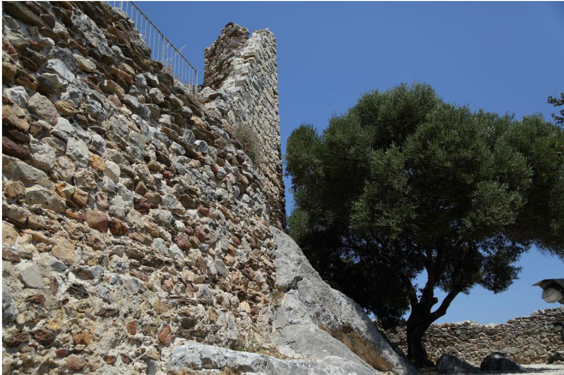
Fig. 4 - Detail of the walls built directly on the rock (photo by Unicity S.p.A.).
