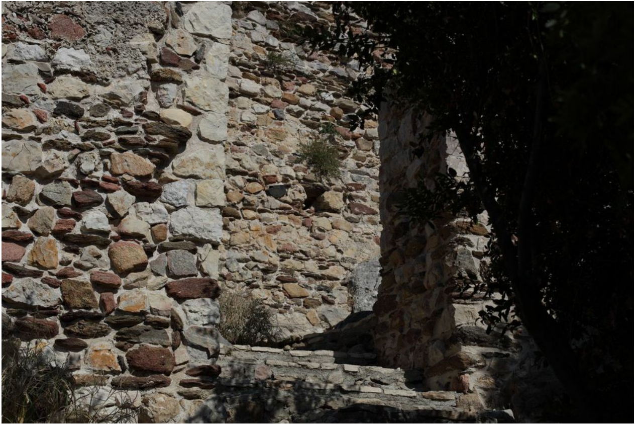
Fig. 4 - Access to the second ring walls (photo by Unicity S.p.A.).
