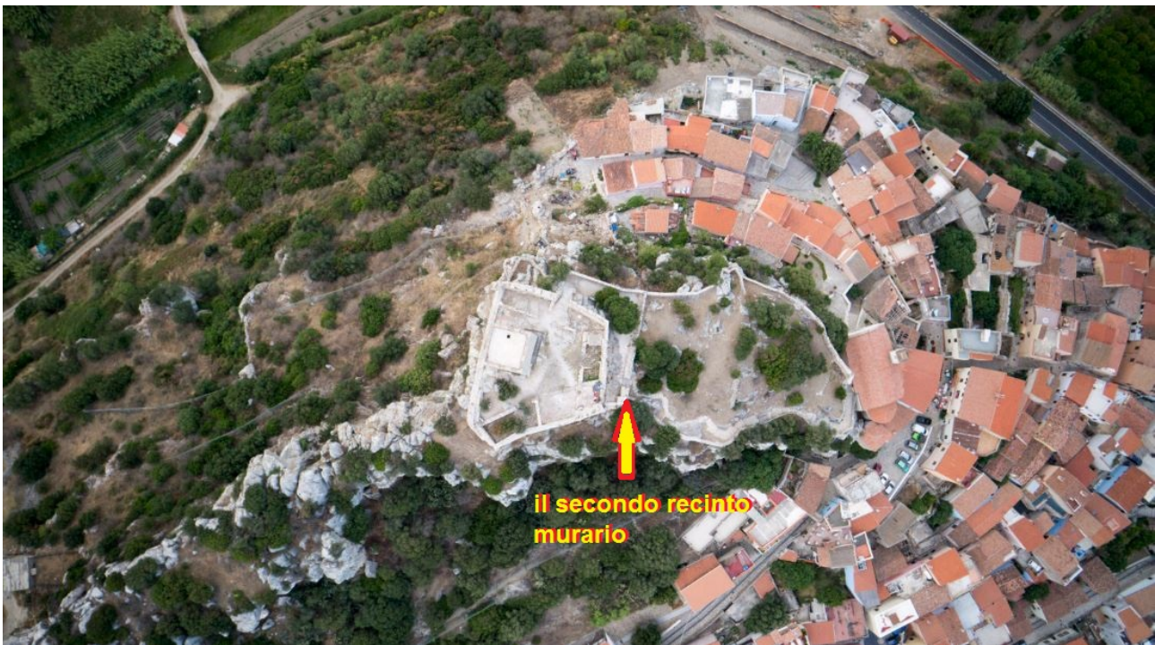
Fig. 1 - The fortress of the castle della Fava which shows its secondary boundary wall (Reconstruction by M. G. Arru, photo by Unicity S.p.A.).
