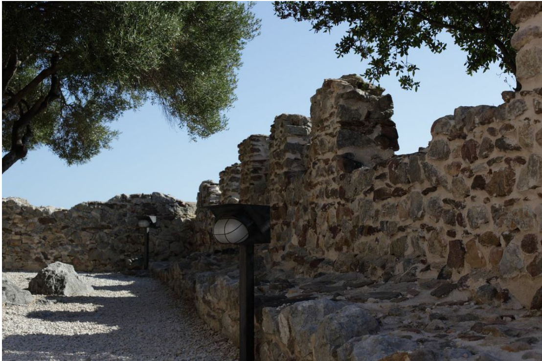
Fig. 2 - Guelph-type battlements visible on top of the ring wall (photo by Unicity S.p.A.).
