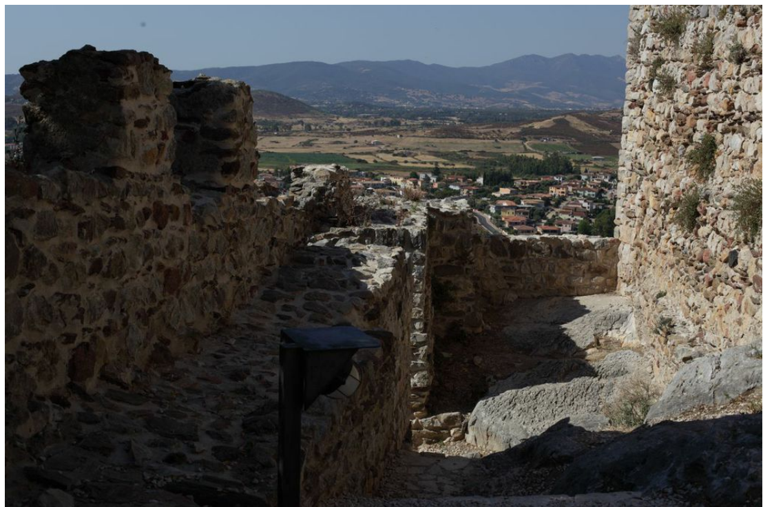
Fig. 3 - The outer wall is built directly on the rock, following the gradient of the slope (photo by Unicity S.p.A.).
