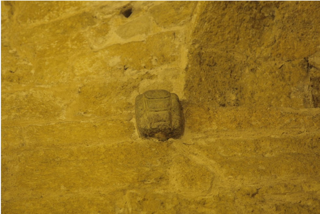
Fig. 8 - Sant'Antioco, the dome's corbel shaped as a tortoise shell (photo by Unicity S.p.A.).
