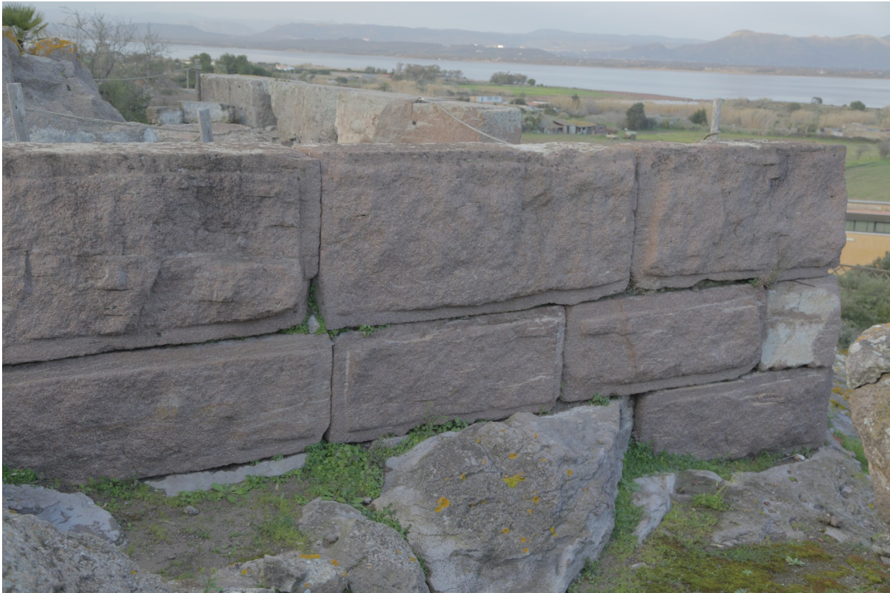
Fig. 2 - Detail of large ashlar trachytic boulders, which enclosed the heart of the Tophet ( photo by Unicity S.p.A. ).
