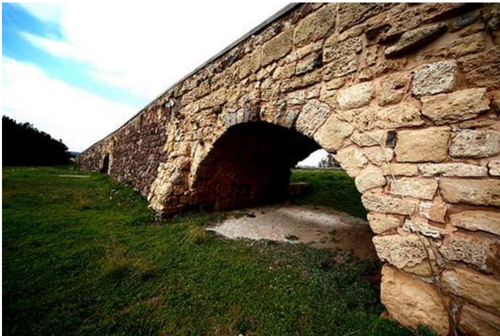
Fig. 3 - Sant'Antioco, bridge built on the remains of a Roman bridge (from https://www.flickr.com/photos/vincenzovacca/8367735306/in/set-72157632483827575 )
