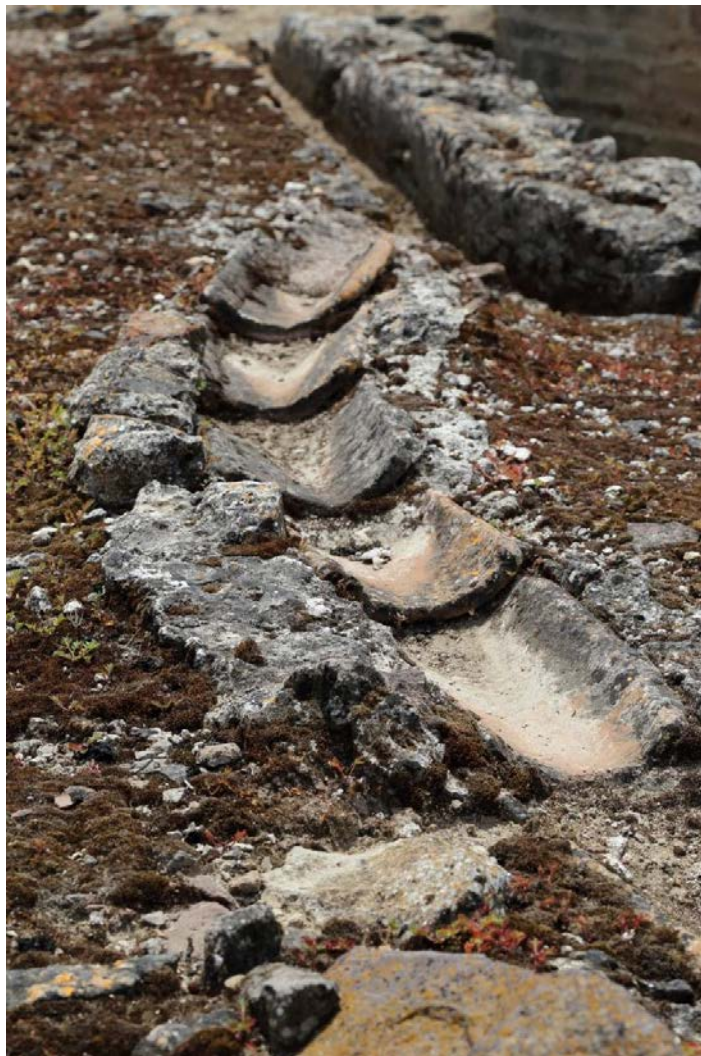
Fig. 1 - Detail of a duct in tiles (photo by Unicity S.p.A.).
