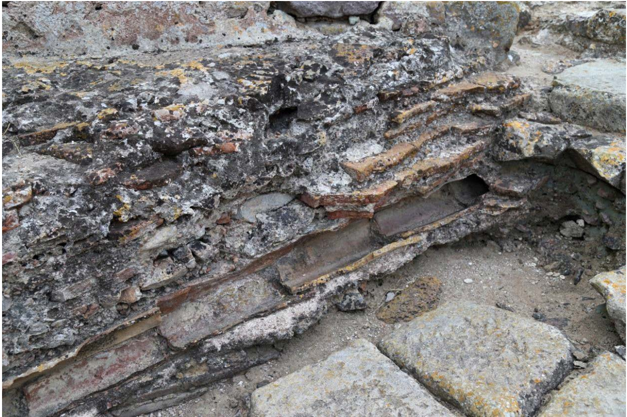
Fig. 3 - Duct originally inside the wall (photo by Unicity S.p.A.).
