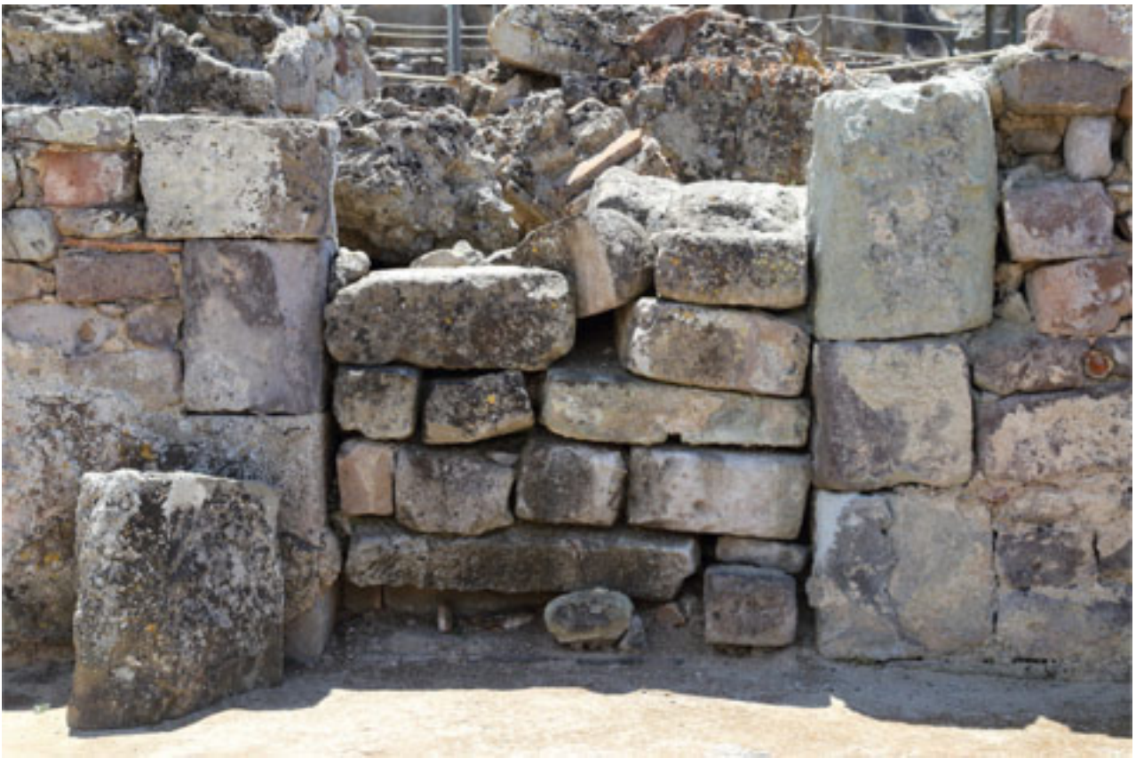
Fig. 12 - The entrance to the frigidarium occluded in the Late-Antiquity period (photo by Unicity S.p.A.).
