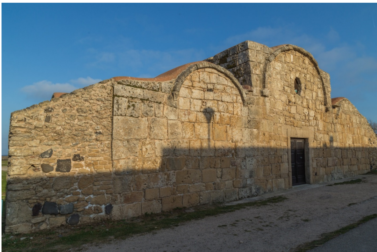
Fig. 6 - Façade of the church of San Giovanni (photo by Unicity S.p.A.)
