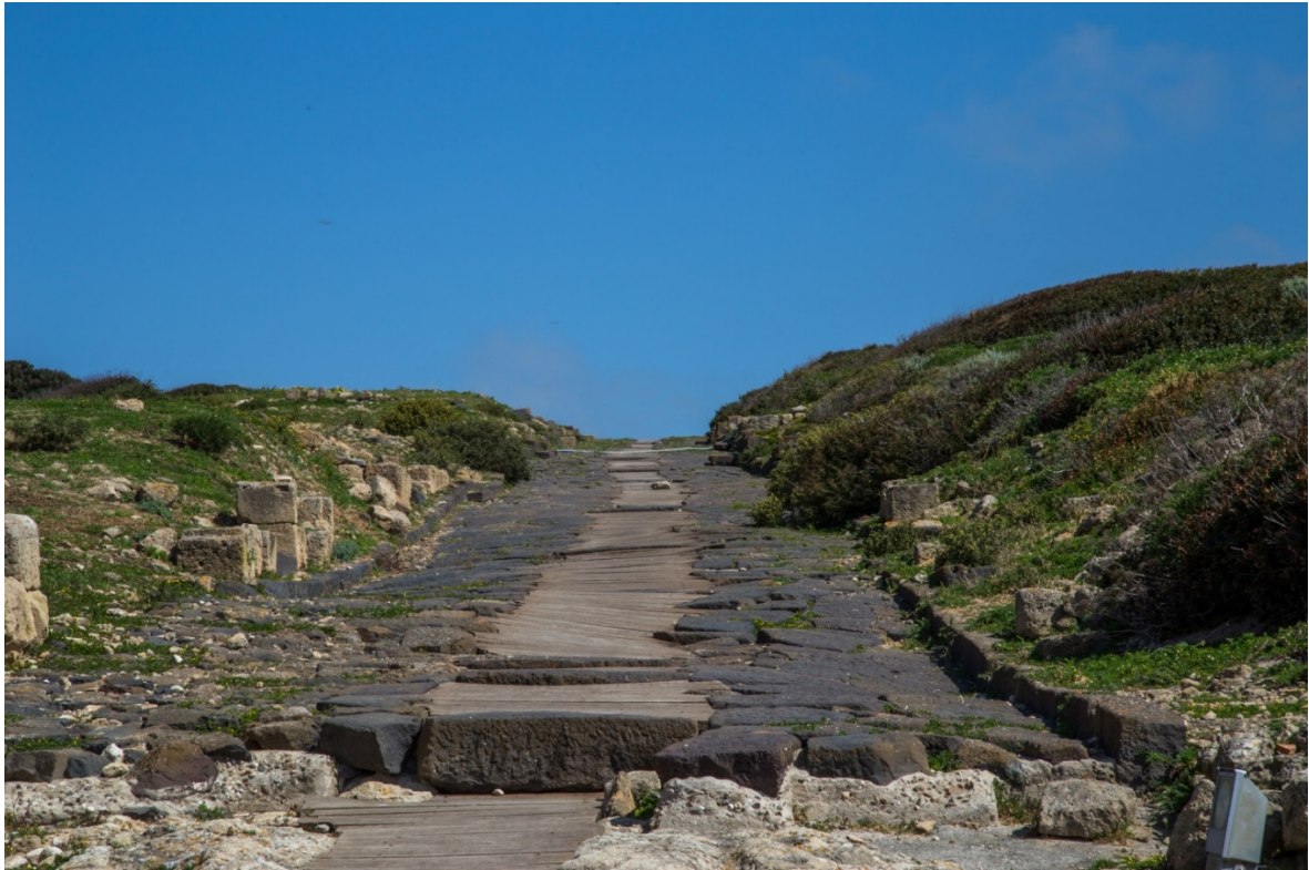
Fig. 8 - Roman road: modern covering in wood in the centre lines the sewer cavity (photo by Unicity S.p.A.)
