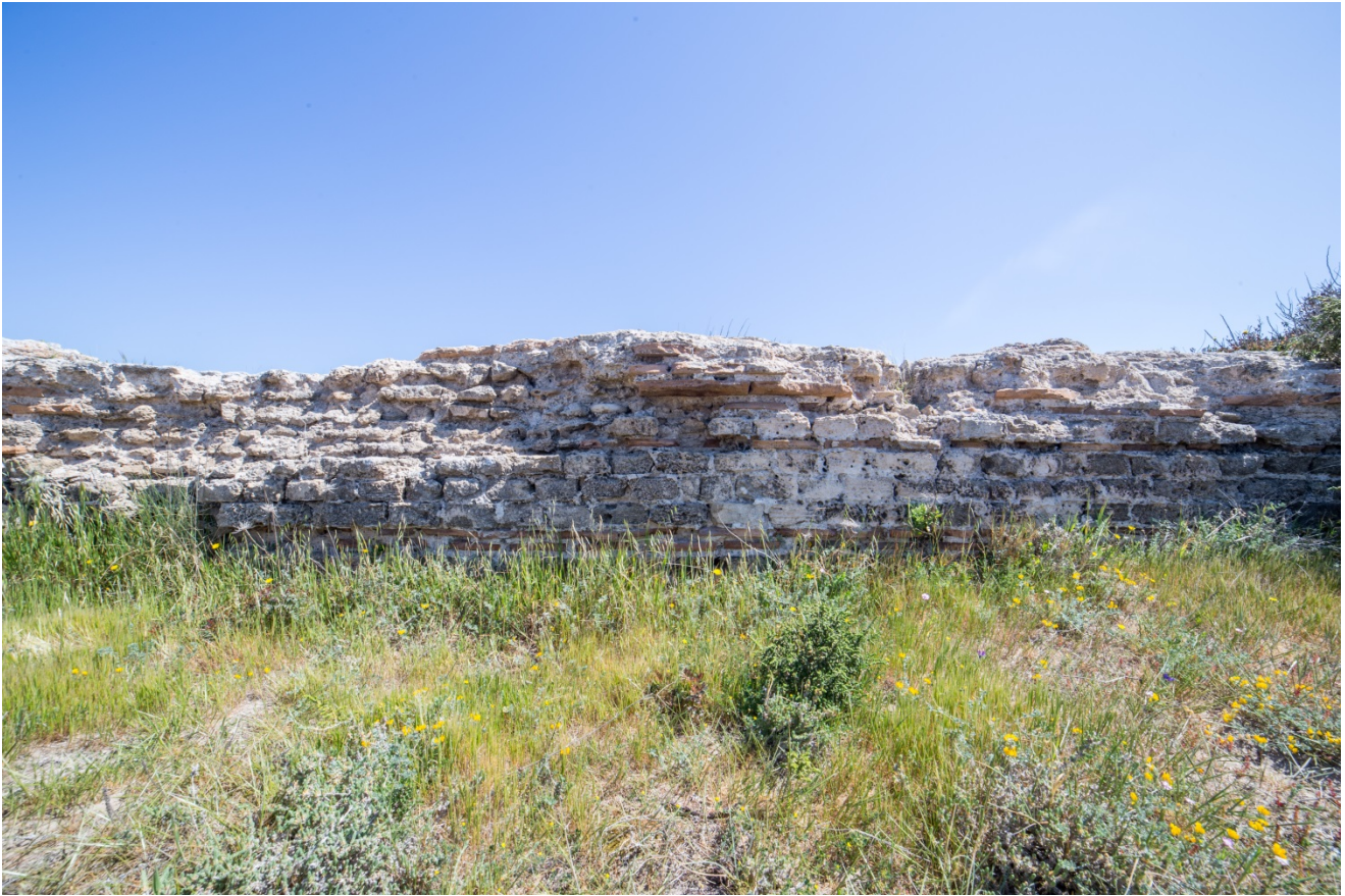
Fig. 4 - The building structure of the aqueduct (photo by Unicity S.p.A.)
