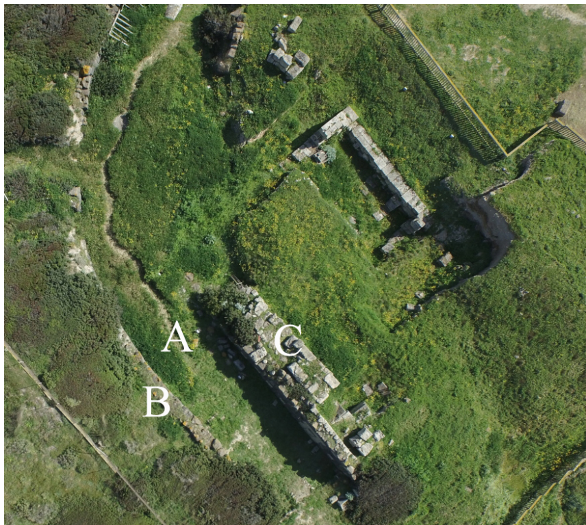
Fig. 1 - Northern fortifications: A) the moat; B) the counterscarp wall; C) the perimeter wall (photo by Unicity S.p.A. Reprocessed by C. Tronchetti)
