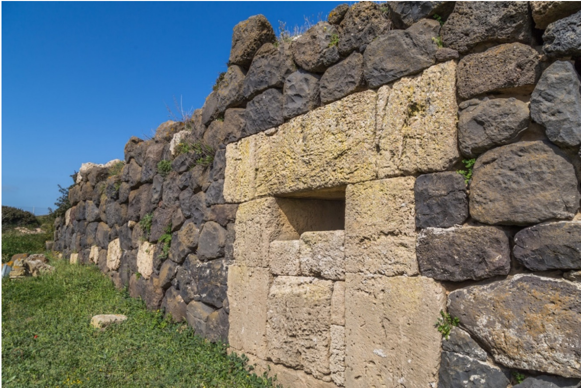
Fig. 2 - The perimeter wall of the fortifications, with the postern blocked up at a later date (photo by Unicity S.p.A.)
