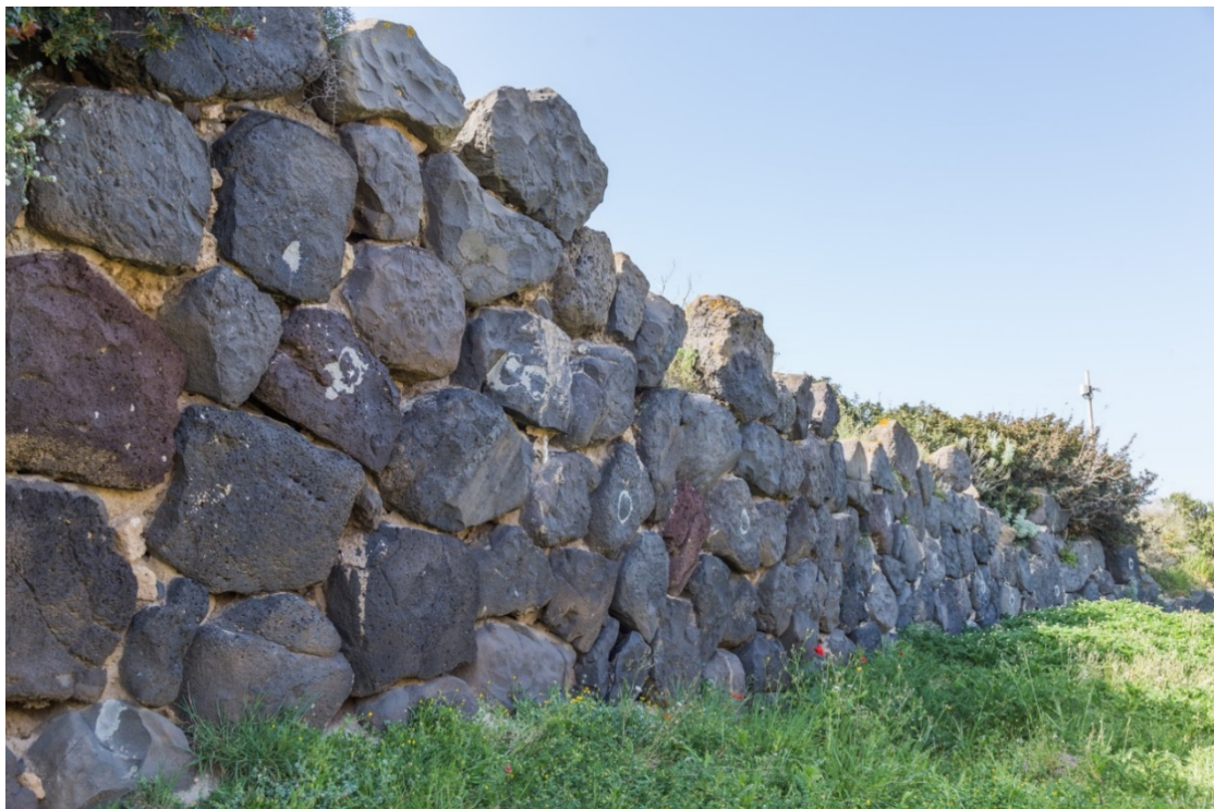
Fig. 3 - The fortification's countescarp wall (photo by Unicity S.p.A.)
