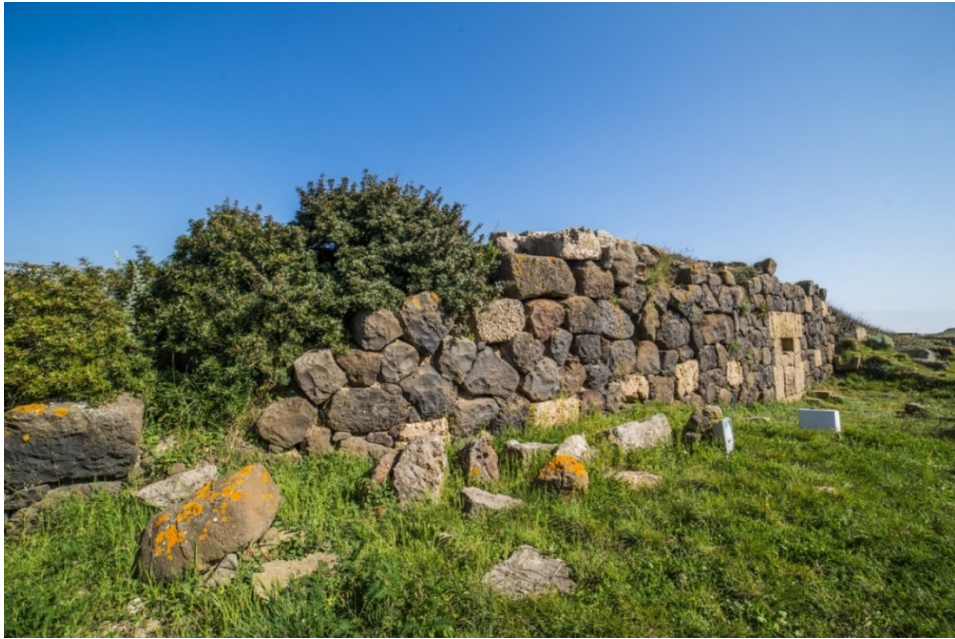
Fig. 4 - The basalt perimeter wall with smooth sandstone blocks (photo by Unicity S.p.A.)
