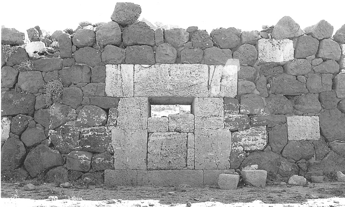
Fig. 8 - A blocked postern in the Tharros moat (Cagliari and Oristano Archaeological Authority)
